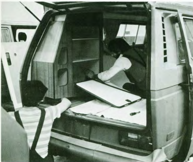
Installation of custom paneling.
